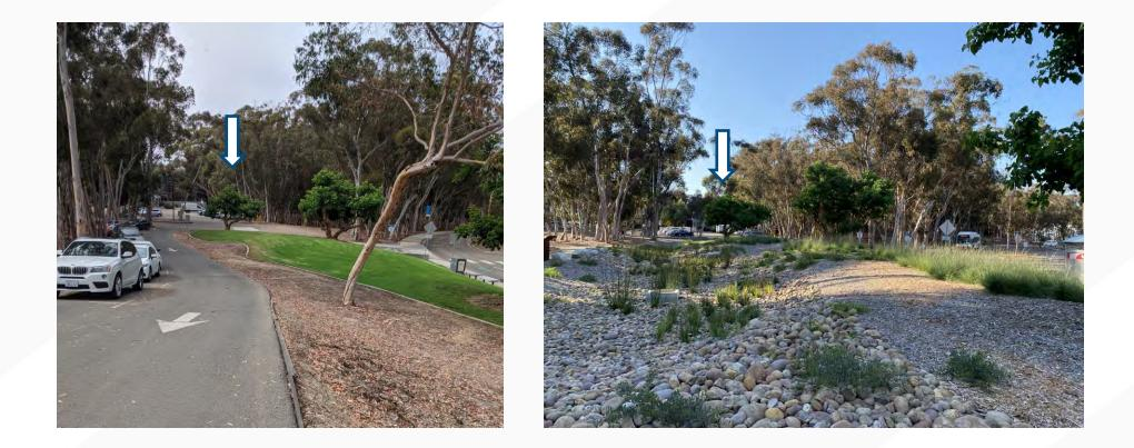
The campus replaced an asphalt road used for parking and a turf area with a stormwater treatment detention basin and drought-tolerant landscaping.
